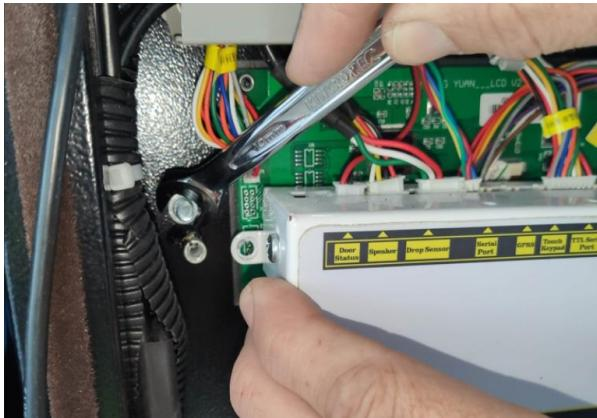
Step #3 – Find a suitable location for the new Perspex Protector so it covers the Nayax Unit, mark the holes with a marker pen, drill the required holes and attach using the supplied bolts.
