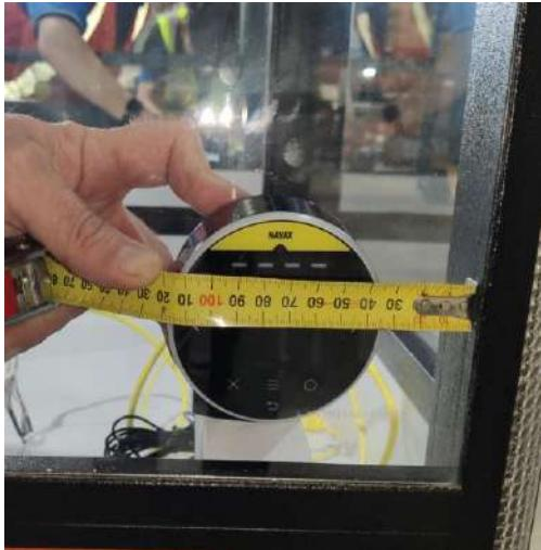
Step #2 – Tilt the positioned unit and mark the centre of the hole with a vivid marker.
