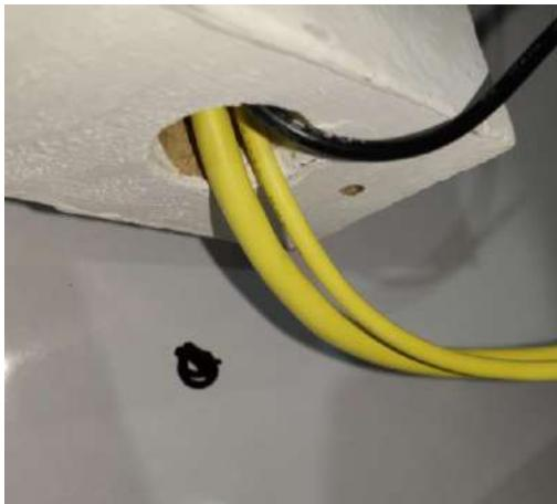
Step #3 – Using a 30mm drill bit drill the hole you have marked.
